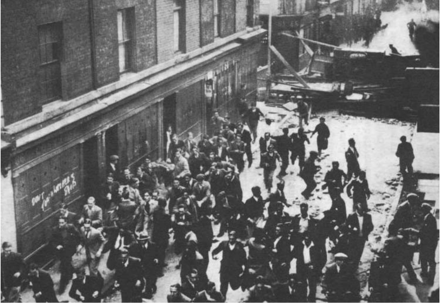
Cable Street, 1936. No platform for fascists - then and now!
